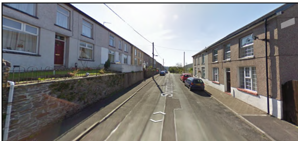
Fig. 5 - Sunnyside Streetscene (looking southwards)
